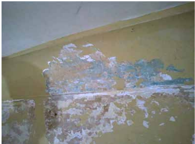
C18 paint finishes revealed
